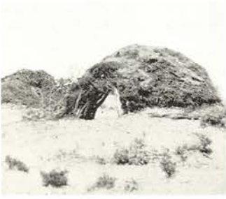
Aboriginal camp of low domed huts made of leaves and sand placed over a wooden frame to effect good insulation against the extremes of the desert climate.
